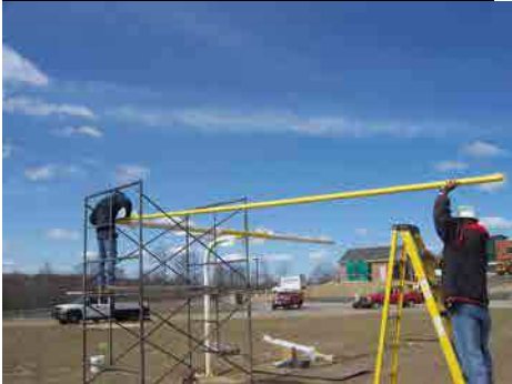
Attaching top upright to end fitting. See Figure 3
