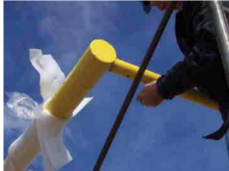
Attaching top upright to end fitting. See Figure 3
