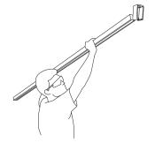
Slide 96" Slotted Track through the Channel Trolley Supports so that the centers of the brackets are 2 feet from the end of the Slotted Track
