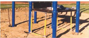
The second method is to pre-install the (4) deck clamps so that there is 42 ½4" between the holes in the deck clamps. Use a level and a marker to make sure the clamps are level to each other. Then place deck onto clamps and bolt. This method works but is less stable than the first method. The deck and posts will stabilize more as you add components Pre-install deck clamps and level.
