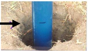
Install red plastic end caps on post bottoms. Install 10" square plywood squares in bottom of holes. Since your holes are 12" diameter and posts are centered in holes you have approx. 3.5" all around the post. Block the posts into center of holes when posts are on bubble. Use scrap lumber and wedges to solidify the posts in their holes as you level the posts. Re-blocking may be necessary at times in order to achieve level. You may also have to widen your holes if they are not dug center.
