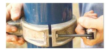
Use magnetic levels on all sides of the round posts. Always adjust the posts into level by gently bumping the bottom with a construction bar. Trying to push the posts into "bubble" in the top or middle will throw off your previous work. Adjust the post levels carefully, not roughly.
