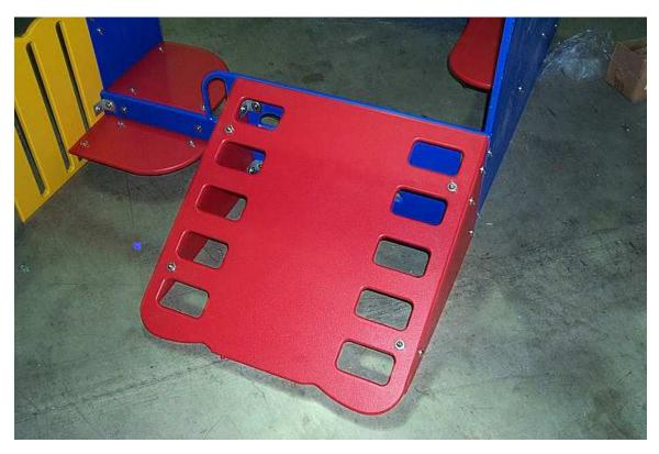
15. Install 8 corner brackets to the 8 remaining holes in the back panel (A) and the front entry panel (D). These holes are located along the top edge and will be used for the roof panels (P).
