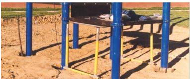
The second method is to pre-install the (4) deck clamps so that there is 42 ½" between the holes in the deck clamps. Use a level and a marker to make sure the clamps are level to each other. Then place deck onto clamps and bolt. This method works but is less stable than the first method. The deck and posts will stabilize more as you add components Pre-install deck clamps and level.
